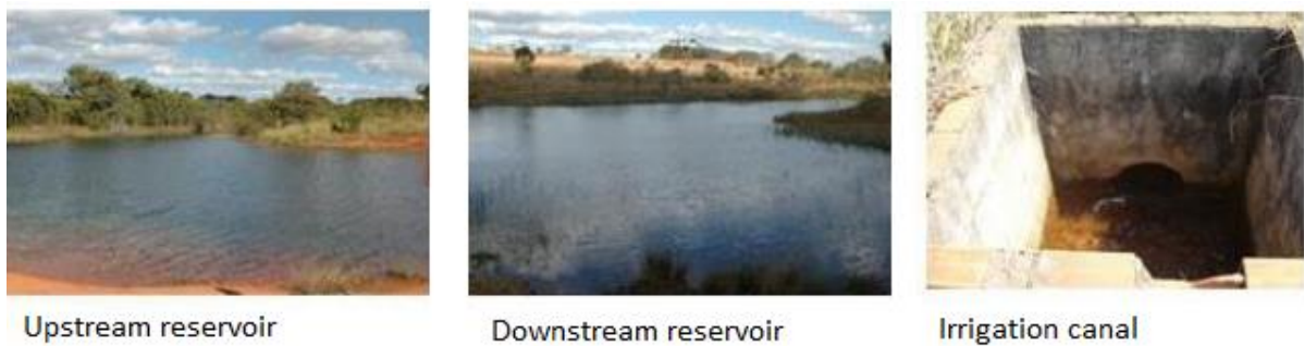
Figure 34. Images of the reservoirs in the Buriti Vermelho watershed and one of the two irrigation canals (Rodrigues & Torres, 2015)
