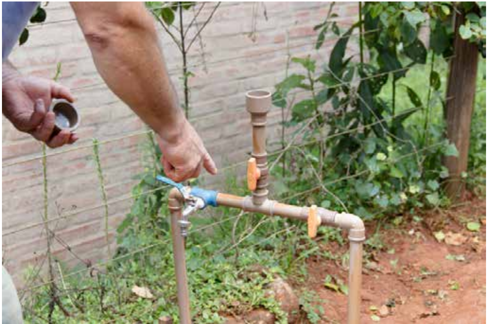
Figure 11. Easy to assemble and low cost chlorine dispenser.
