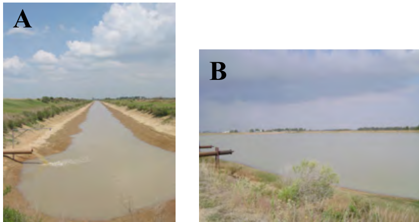
Figure 2. Tail-water recovery ditch (A) collects irrigation and rainfall runoff from fields. This water is pumped to a 15-ha reservoir (B) for future use.
