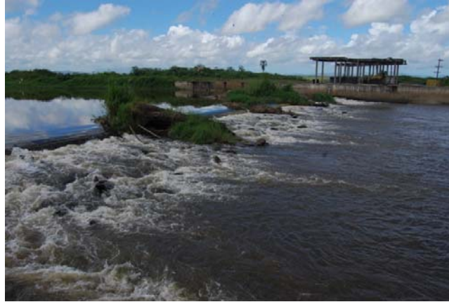
Figure 21: Water diversion structure at the beginning of Imunana channel.
