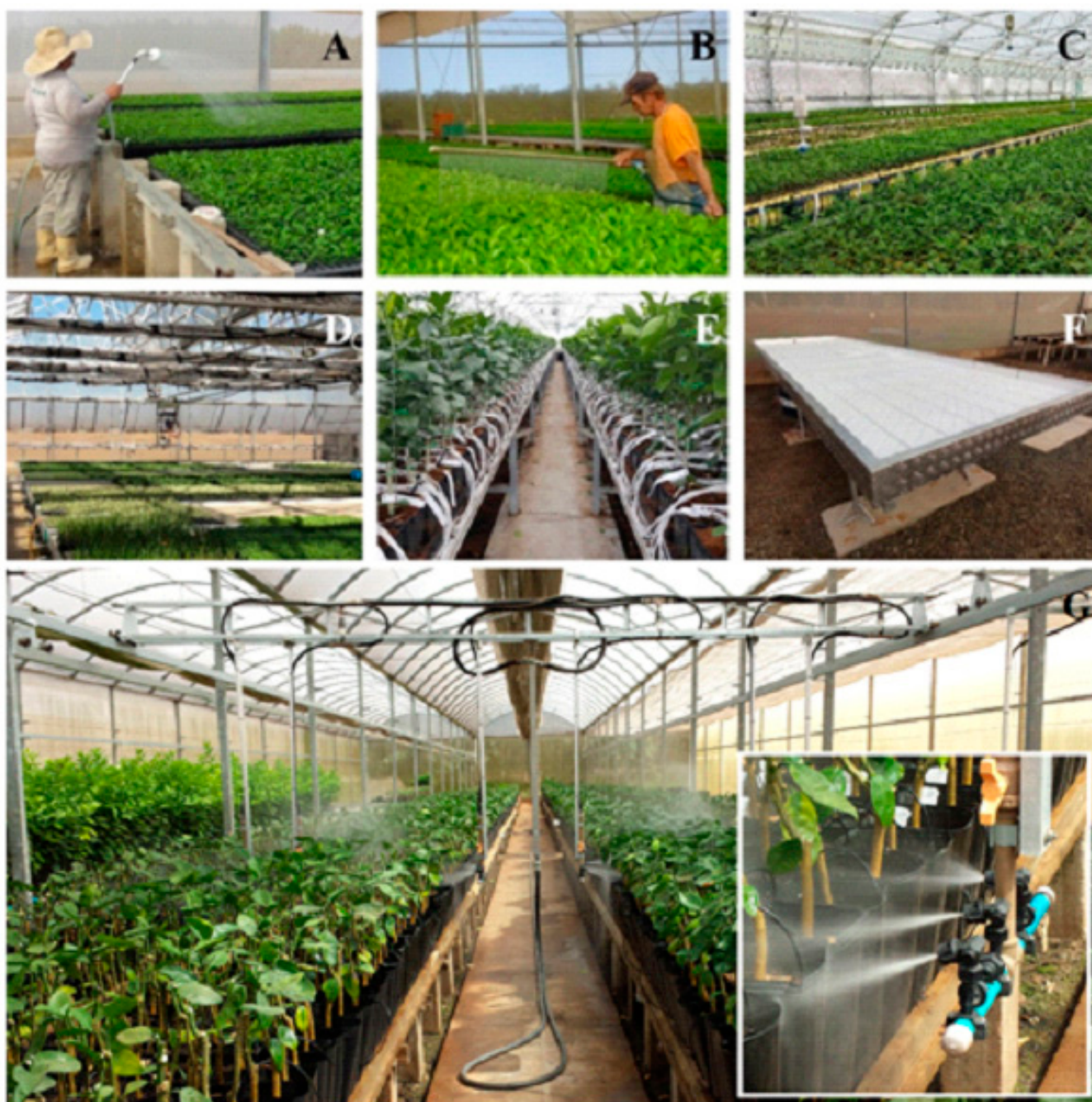
Figure 4. Irrigation systems used in commercial citrus nurseries for the production of rootstock seedlings, nursery trees and budstick in budwood increase blocks: A) shower head, hose nozzle or rain wand (Photo: Rhuanito Soranz Ferrarezi); B) perforated PVC pipes (Photo: Conan Ayade Salvador); C) micro sprinklers; D) spray bars; E) drip system; F) ebb-and-flow subirrigation (Photos: Rhuanito Soranz Ferrarezi) and G) Mobile bar in budwood block (Photo: Sérgio Alves de Carvalho).
