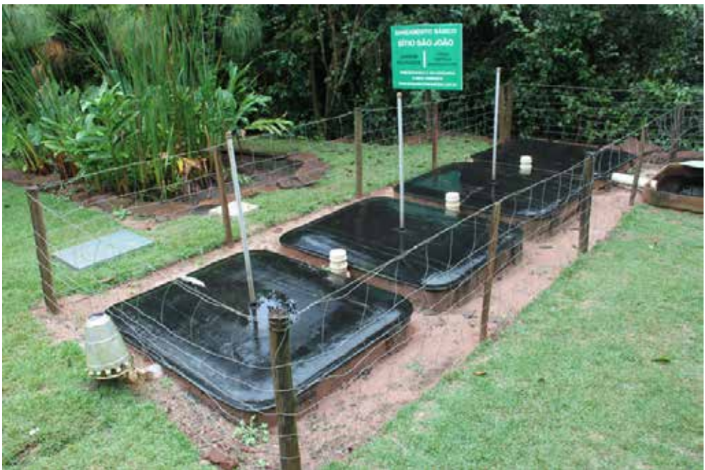
Figure 10. Display of biodigester septic tank for treatment of domestic sewage.
