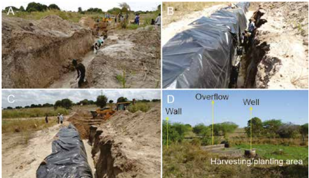
Figure 2. Opening of the dam of the underground dam (A); placing the plastic in the ditch by waterproofing the wall (B); ditch closing (C); underground dam ready, with wall, well, bleeding and planting area (D).
