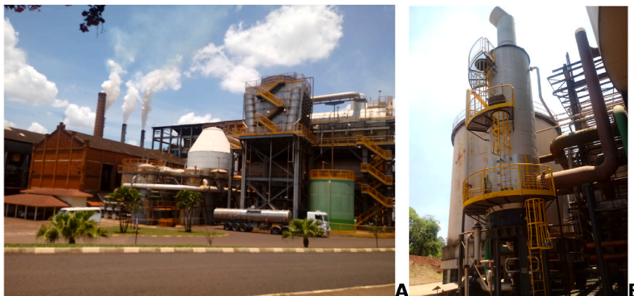
Fig. 2. An ethanol plant (A) with its chimney of carbon dioxide emission from fermentation vessels (B). This plant is located in Araraquara region, São Paulo State, Brazil. Credit: Silvio Vaz Jr.
