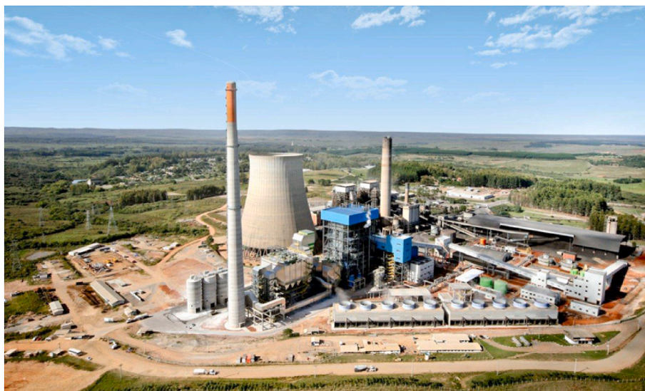
Fig. 1. A thermoelectric plant for energy generation. This plant is located in Candiota, Rio Grande do Sul, Brazil. Credit: Eletrobras.
