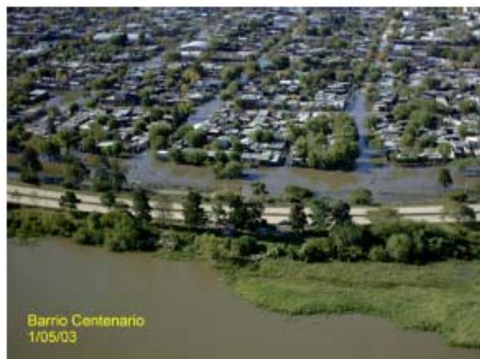
Figure 7 - Flood in West portion of Santa Fe city, April-May 2003 (Source: Paoli, 2004).
