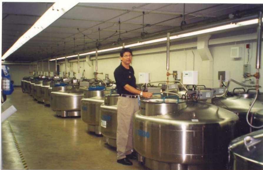
Figura 3. Nacional Center for Genetic Resources Preservation – NCGRP, Ft. Collins, CO, U.S.A. Criopreservação de germoplasma – sementes, a -150^{\circ}\text{C}
