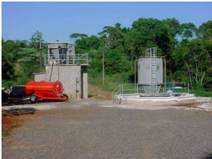
Figure 2. Compact unit designed for swine manure treatment installed at Embrapa Swine and Poultry, in Concordia City, Santa Catarina State
